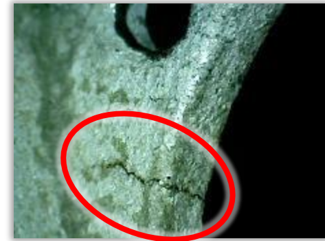
Arcing contact failure mode
