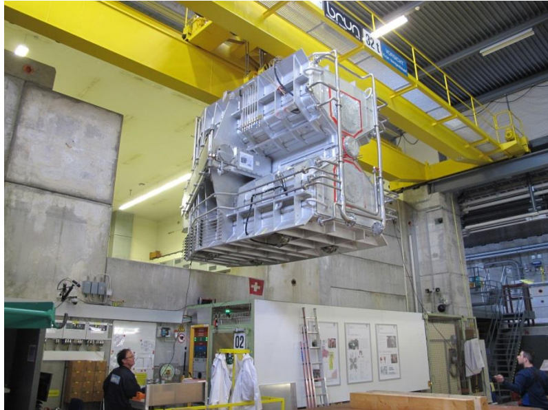
Bringing the new resonator into the injector 2 bunker
