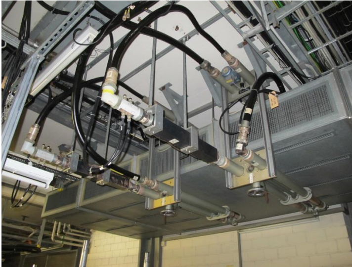
Matching network for 2 x 8 kW/150 MHz combining
