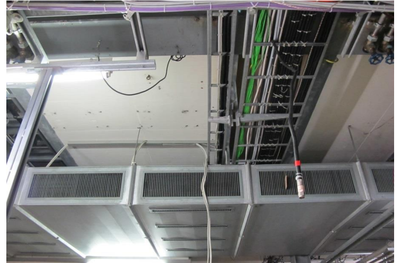
rf-cables, \lambda/4 transformers and phase shifters were removed
