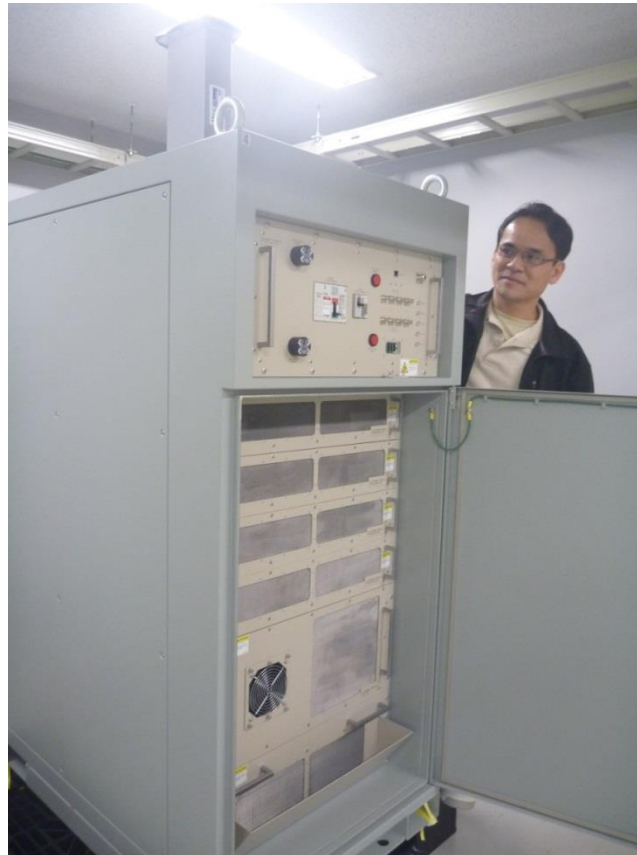
The R&K 1.3 GHz SSA Rack for LCLS II
