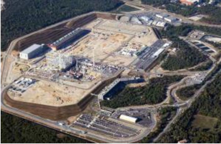
Cadarache, France: building site
