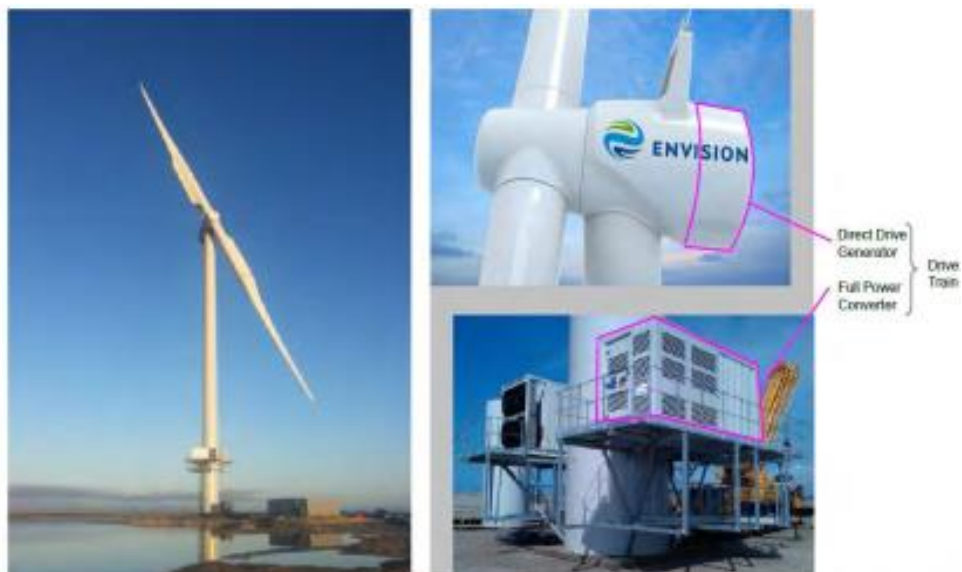
Fig. 1: Envision GC-1 turbine (E128-3.6 MW) installed Thyboren, Denmark. EcoSwing will replace pink parts by an HTS generator and an innovative power converter.
