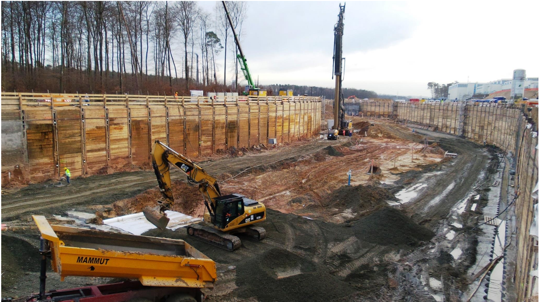
Excavation 1st section of SIS 100
