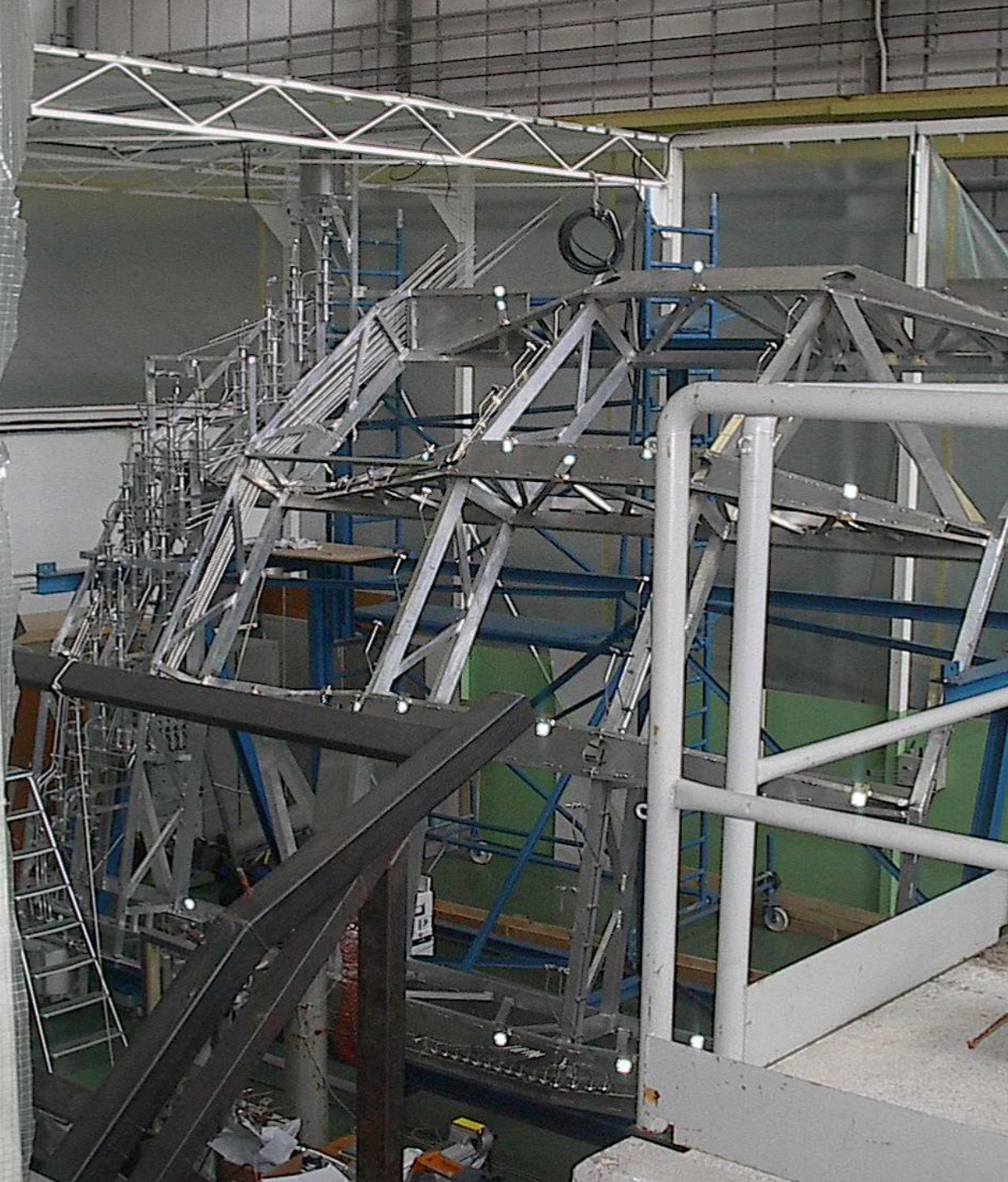
HMPID support structure (incl. services for liquids and gas)
