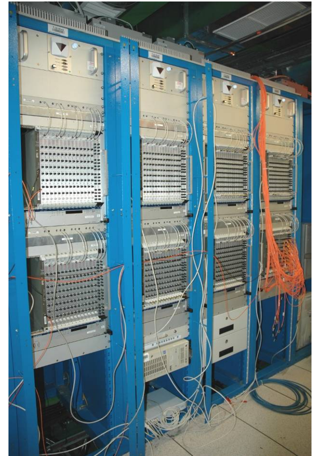
LAr barrel ROD system in USA15
