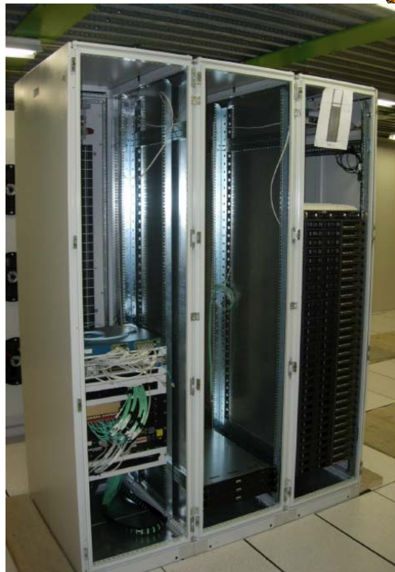
The first full HLT rack in the SDX1 HLT/DAQ room at the Pit-1 surface
