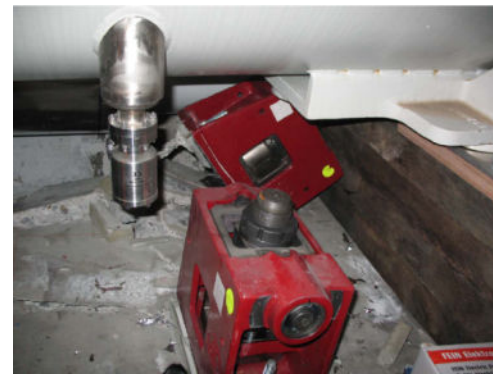
Collateral damage: ground supports
