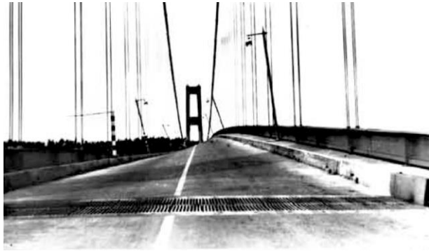
Wrong way to use resonances: Tacoma Narrows Bridge example
