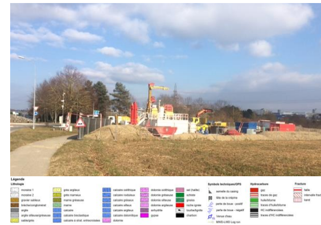
Geothermal site investigation in Satigny 2017/2018 (500m deep)
