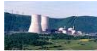
Nuclear Power Station
