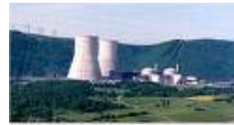
Nuclear Power Station
