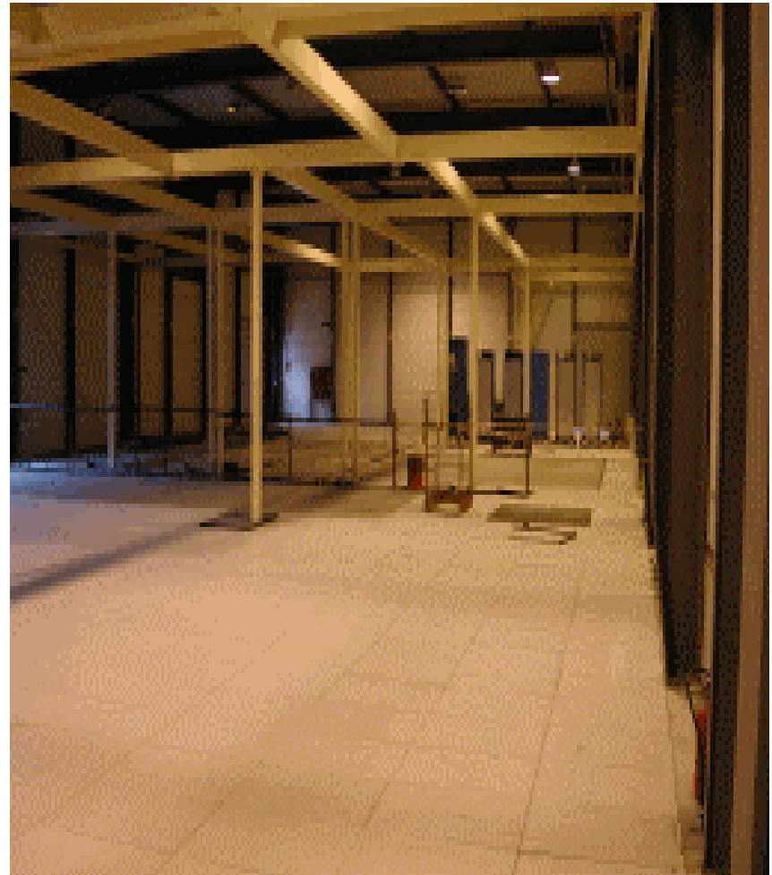
ID clean room facility under construction near the surface building at pit 1
