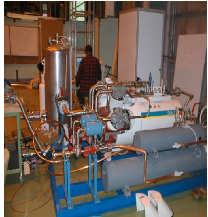
Compressor of the evaporative phase-II Pixel and SCT cooling set-up
