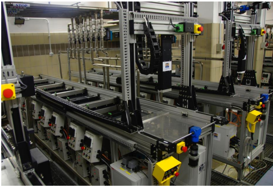
Lab 1, below-ground floor
