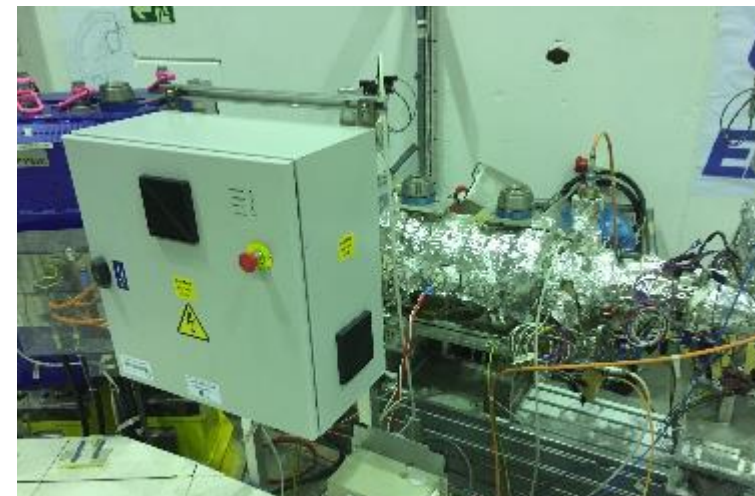
Fast deflector at CERN in ELENA
