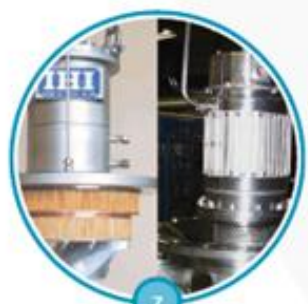
7 CRYOGENICS 2 new large 1.9 K helium refrigerators for HL-LHC near ATLAS and CMS
