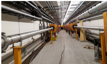
installation of ToF cable along H2 beam line, Feb 2018
