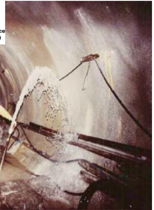
Water inflows during LEP construction
