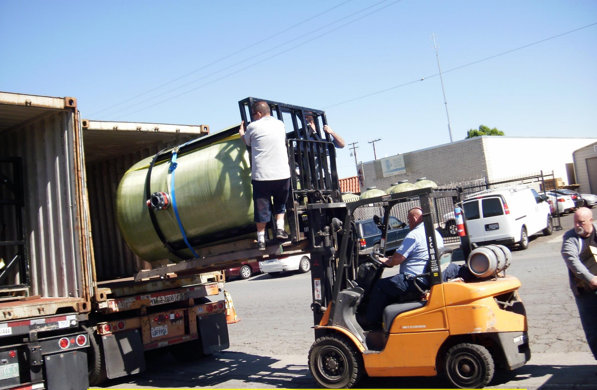
At South Coast Water factory, Santa Ana, CA; Feb. 19 th , 2018
