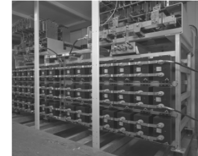
Figure 9: Capacitor Bank, example energy storage for the DVR Israel
