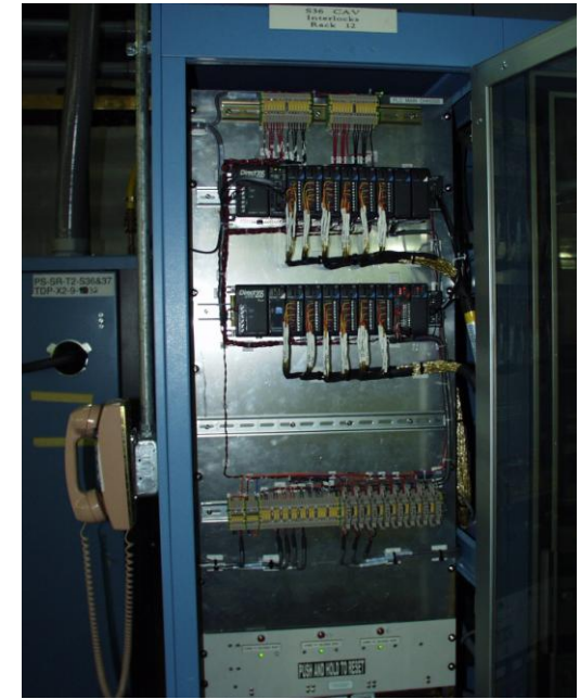
NEW PLC INTERLOCK SYSTEM INSTALLATION
