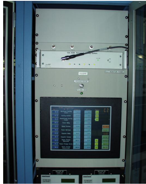
NEW PLC INTERLOCK SYSTEM INSTALLATION
