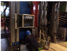
Figure: New muon patch panel
