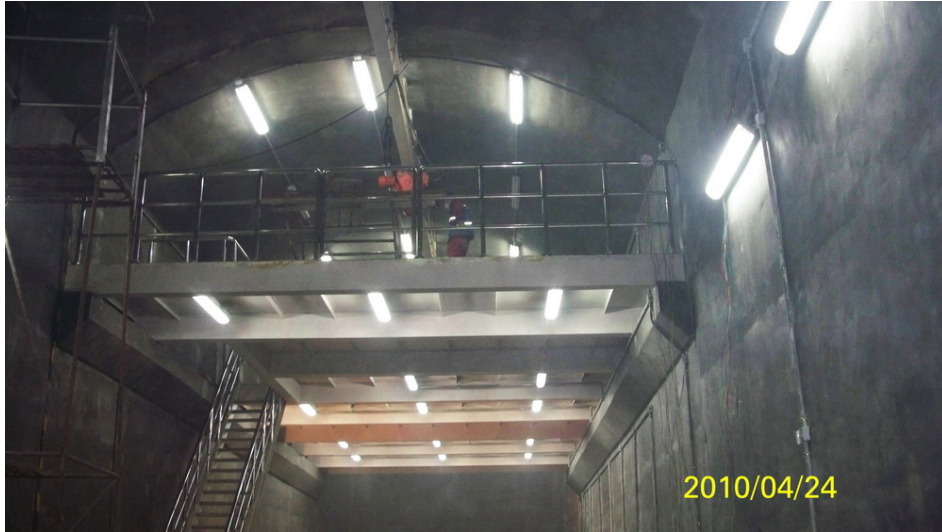
Main hall is ready!
