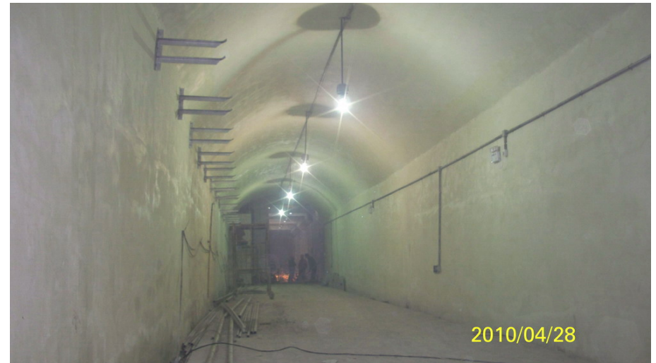
Tunnel to main hall
