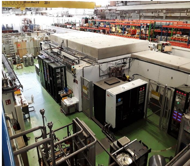
50 MW klystron with pulse duration of 1.2 \mu s
