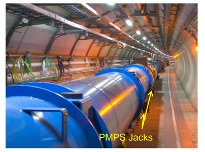
LHC Superconducting dipole magnets supported on Indian PMPS jacks in tunnel
