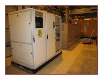
100kV solid state modulator designed, developed and commissioned by RRCAT, Indore, for LINAC 4 cavity tests.
