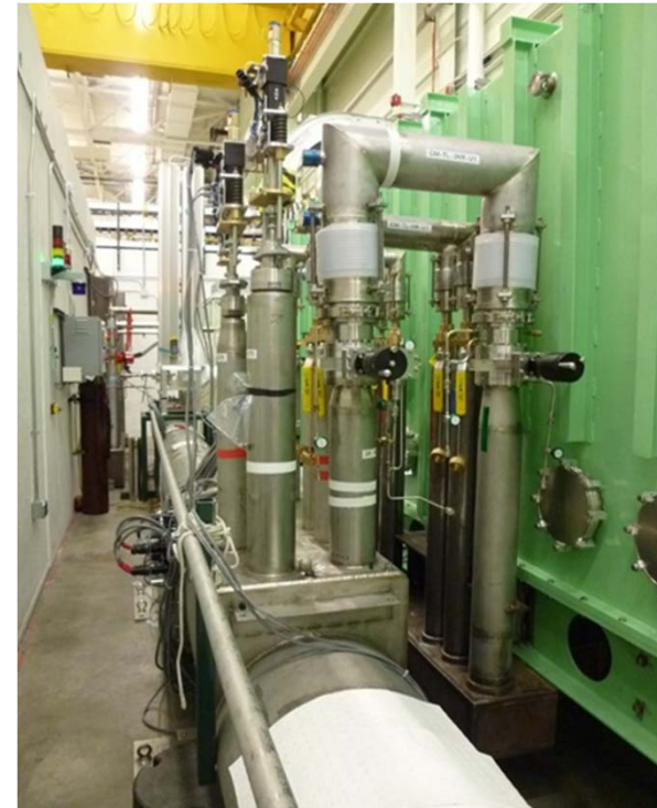
U-Tube connections between CM and cryo Distribution
