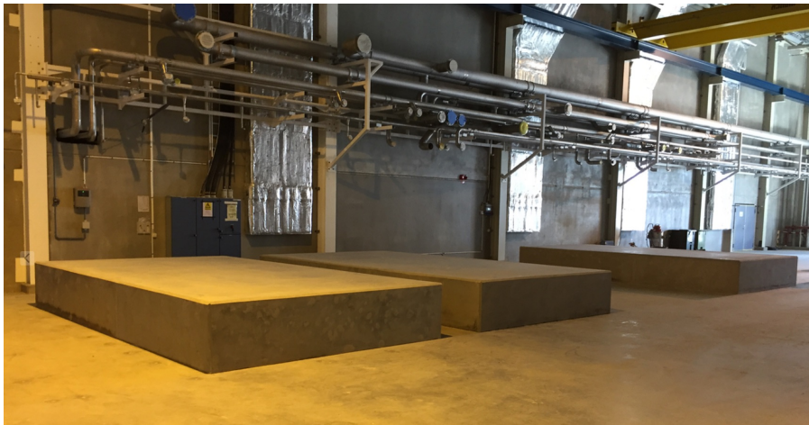
Concrete foundation of compressor skids
