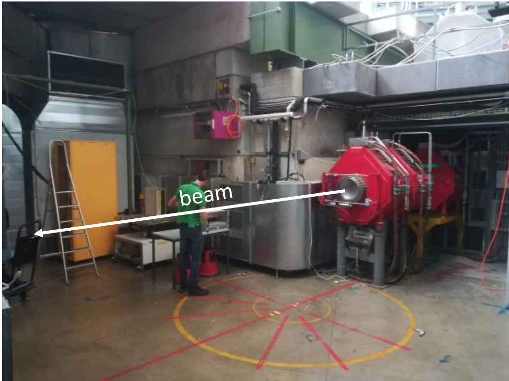
Space available in the area (about 4-5 m along the beam)
