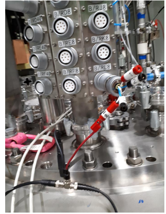
Voltage tap connection
