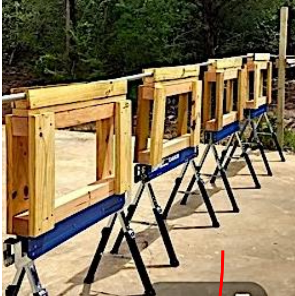
pull straight 150 m cable through sheath tube with loose fit
