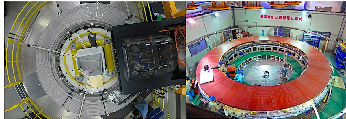
Figure 4. (left) Fabrication proceeding on the first CS module; (right) PF6 sixth double pancake resin impregnated.
