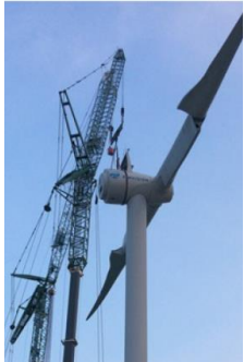
Installed on wind turbine
