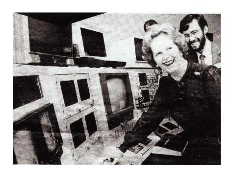
The original ISIS Main Control Room in 1985, shortly after first neutron beam. The user interface was based on the CERN SPS system but was ported to GEC 4000 series computers.
