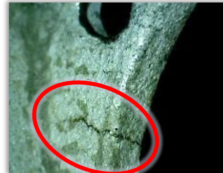
Arcing contact failure
