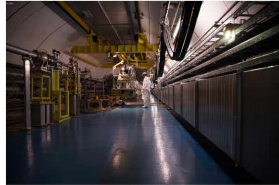
Photographer: Maximilien Brice HRMT27 Installation
