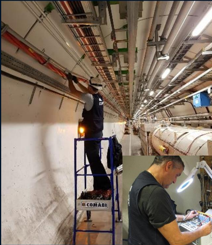
Electrical and cabling installation contract
