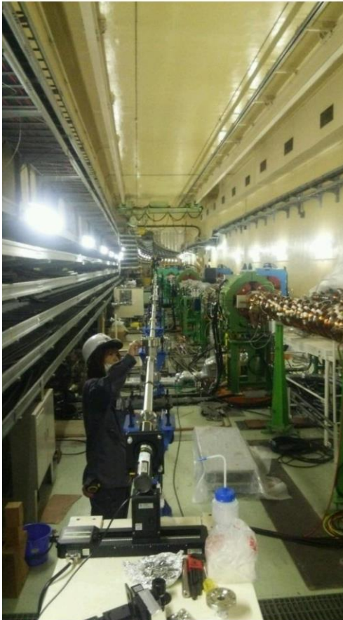
X-ray beam line under construction at LER
