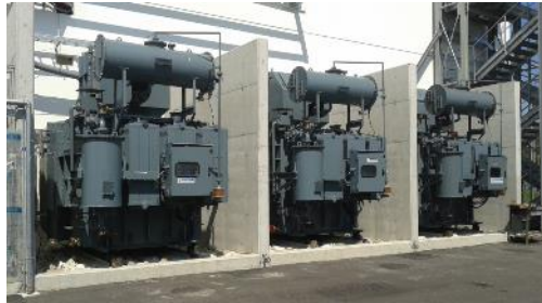
Multi-winding transformers
