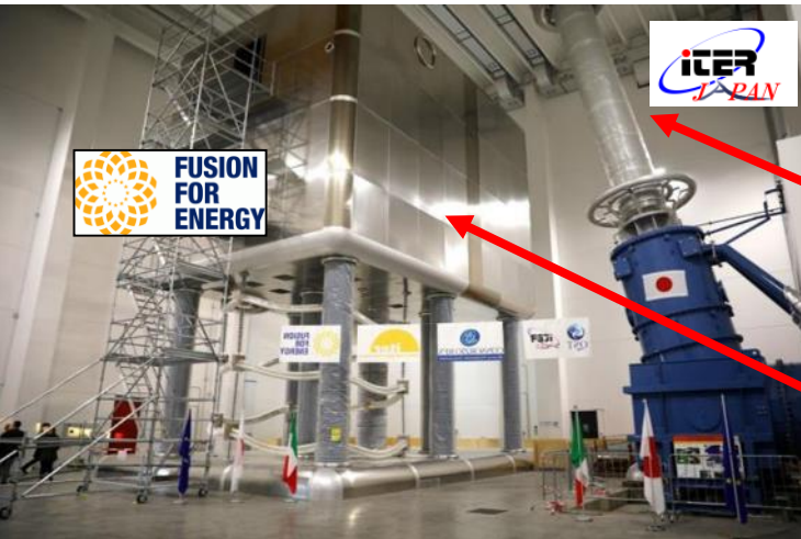
1MV Faraday Cage (hosting Ion Source PSs)
