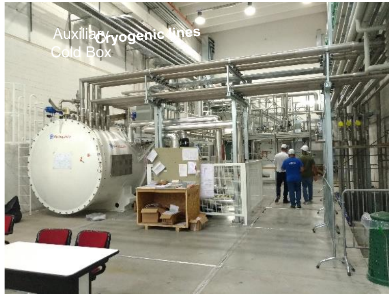
MITICA Cryogenic Plant components and piping inside Building 2 for production and distribution of 4 K SCHe and 80 K GHe
