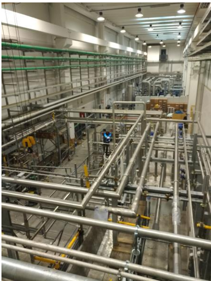
MITICA Cryogenic Plant components and piping inside Building 2 for production and distribution of 4 K SCHe and 80 K GHe
