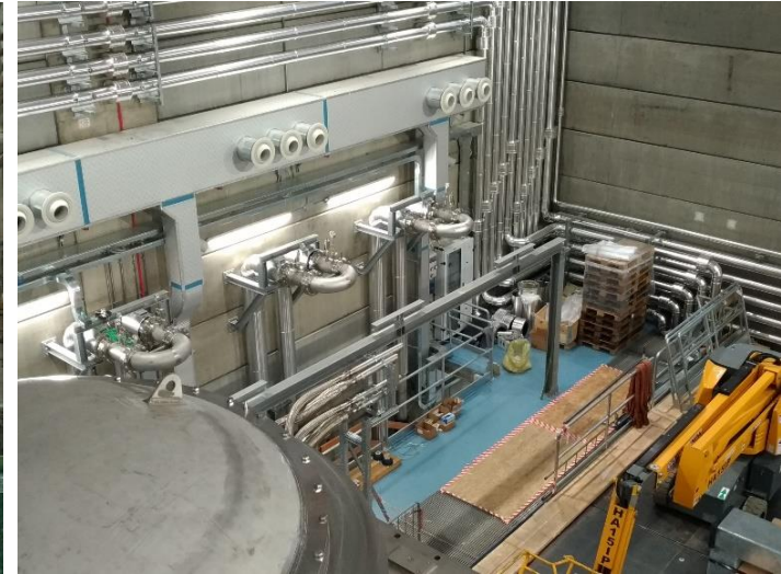
View of Cooling Plant Primary Circuits inside MITICA Neutron Shield
