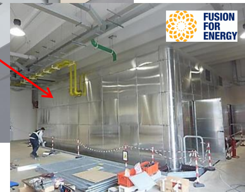
High Voltage Deck (HVD)
