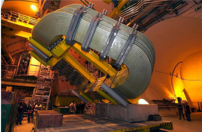
LHCb detector dipole Al coils coil mass 2 \times 25 t power 2 \times 2.1 MW
