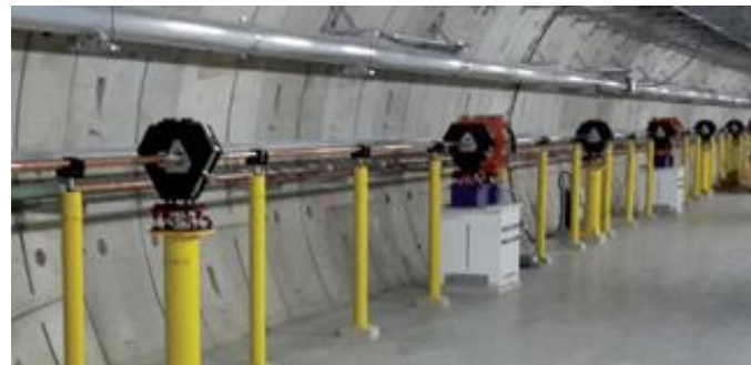
In Line Pumping – XFEL, DESY
