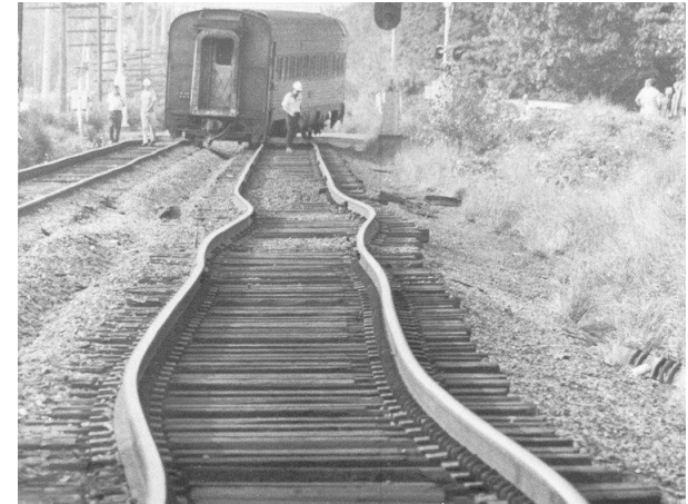
Digression on thermal stresses: Thermal buckling in railway tracks Source: [Business Insider]
