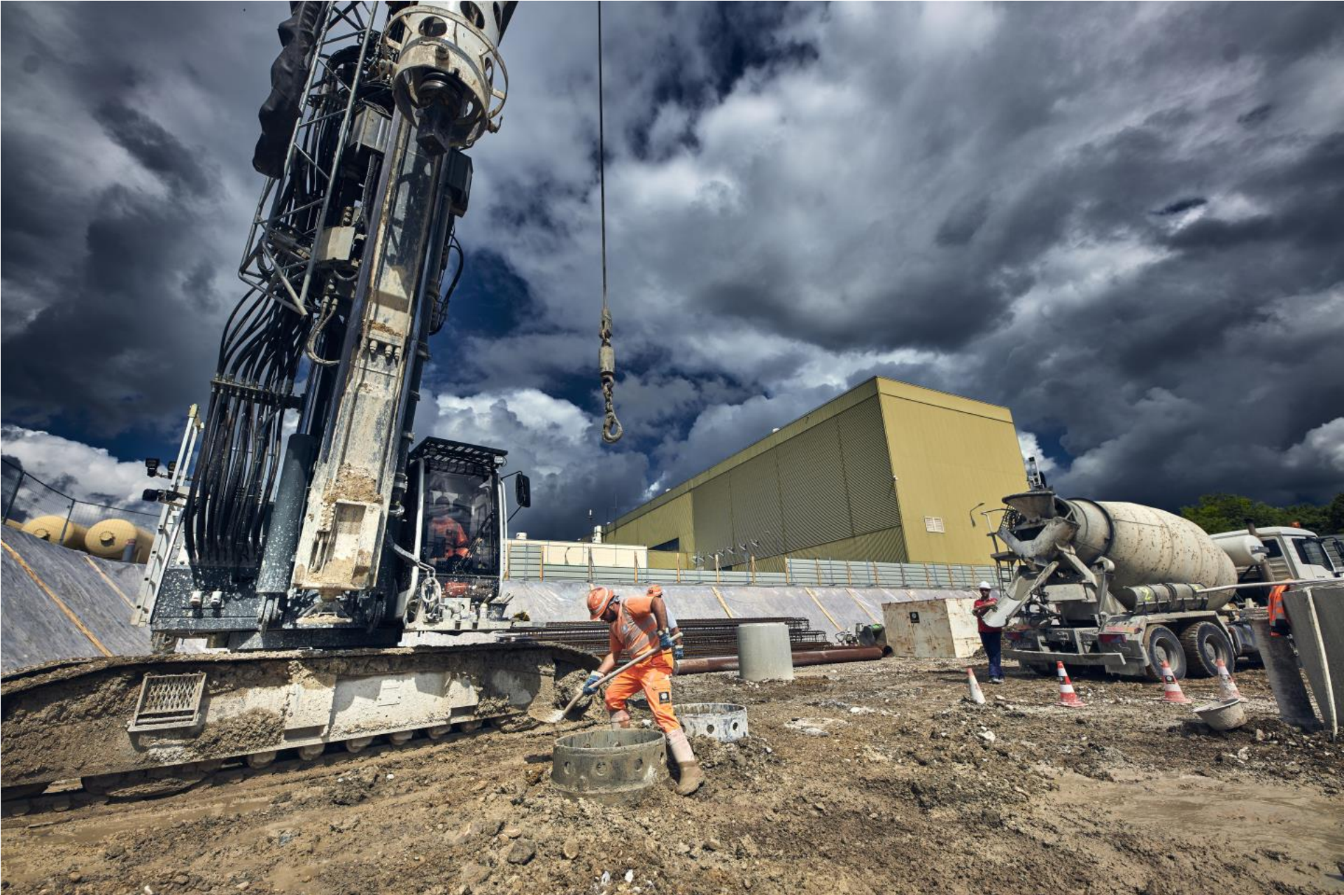
Civil Engineering Pt1 and Pt5 has started
