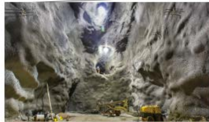
Davis Cavern before lab construction
