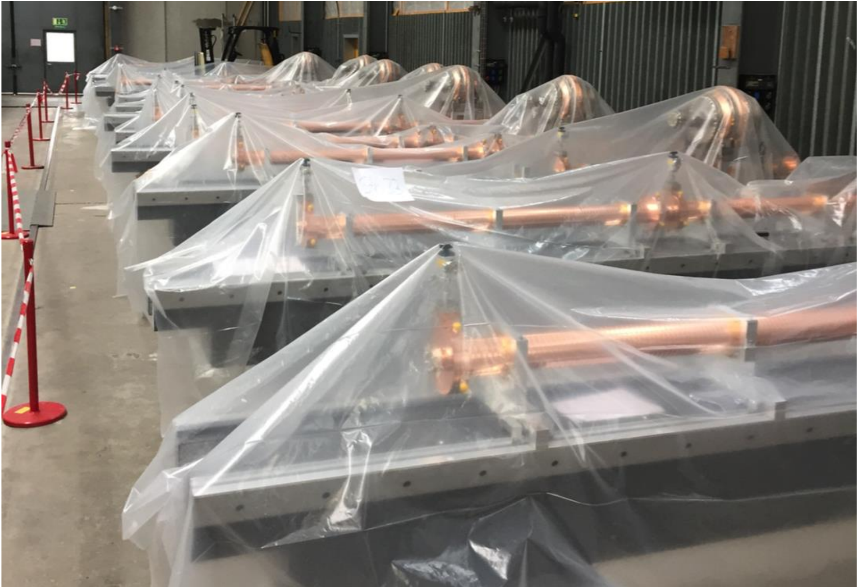
Girders were pre-assembled in a storage hutch
