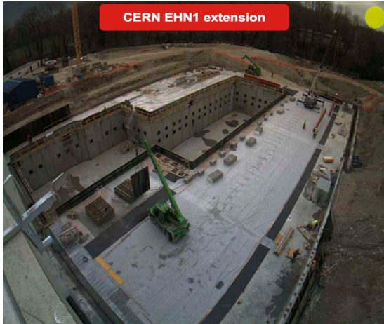
March 2016, construction of EHN1 extension
