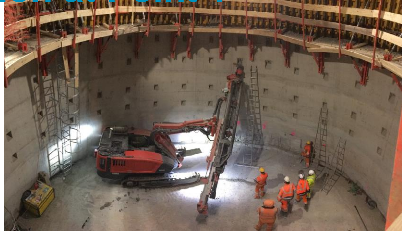
Reinforced concrete ring at the shaft end
