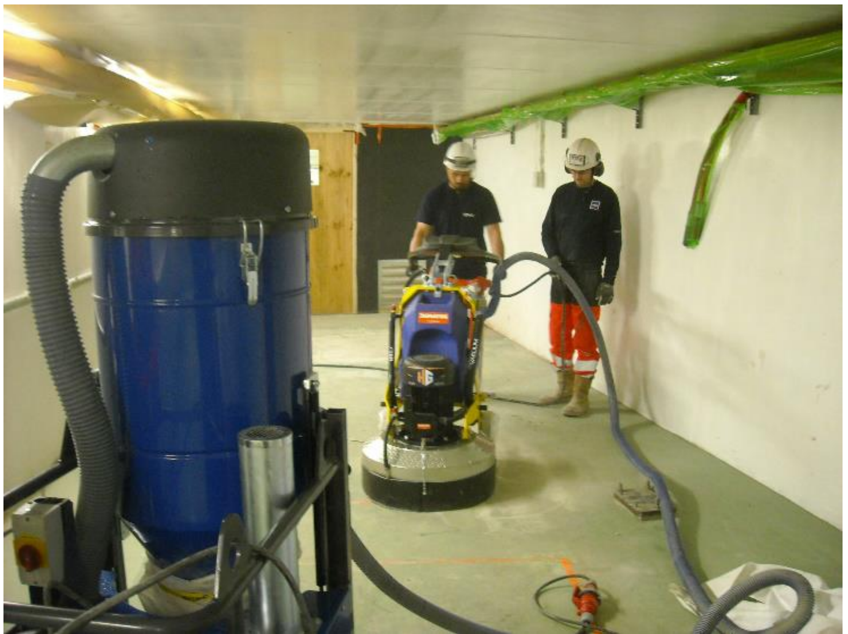
a few views in the tunnel : 4 : grinding the floor
