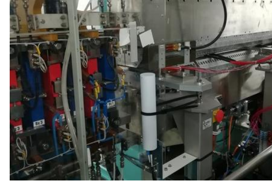
Between undulators Middle of a straight section
