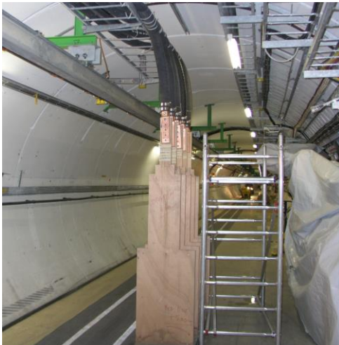
Mockup DFB (LHC installation)
