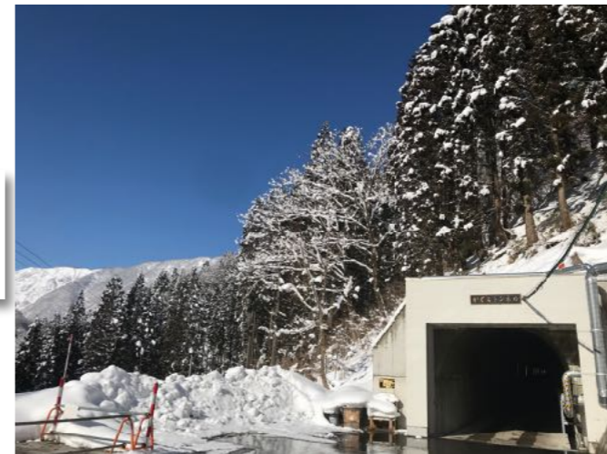
KAGRA Tunnel Entrance
