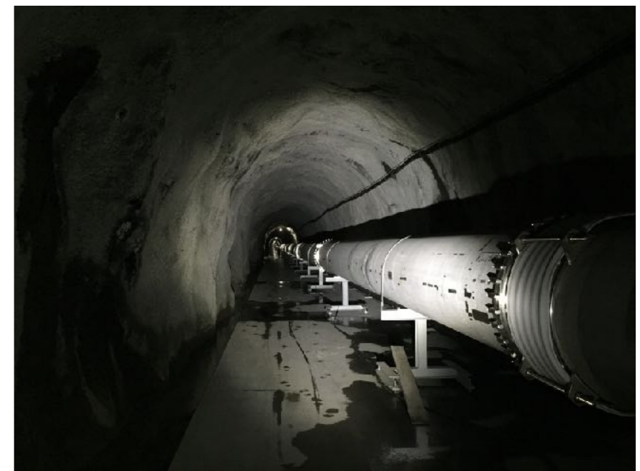
3km beam tube (diameter of 800) Achieved pressure 10^{-6} Pa (req. 10^{-7} Pa)
