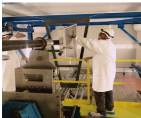
Install new ROC
